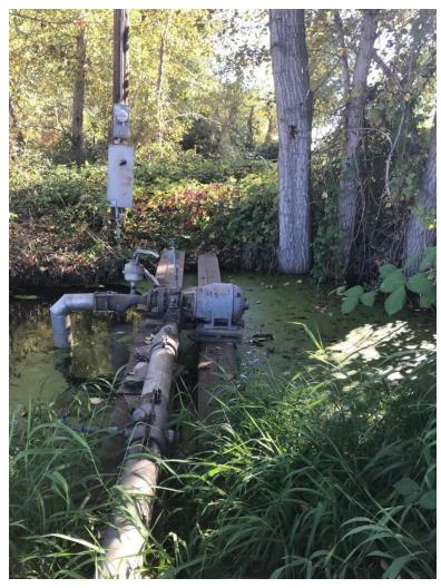
Pump located in West Prong Little Walla Walla River pumps to irrigation ditch
