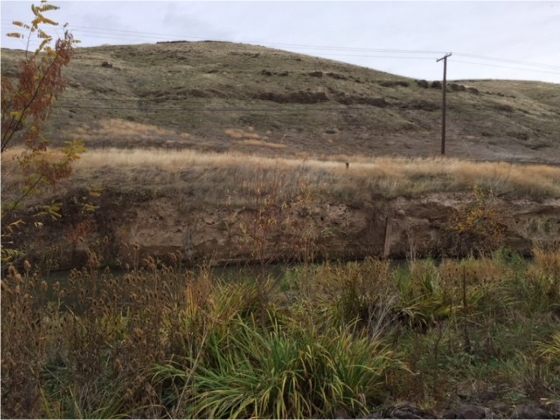
Looking toward east bank where fencing will be installed
