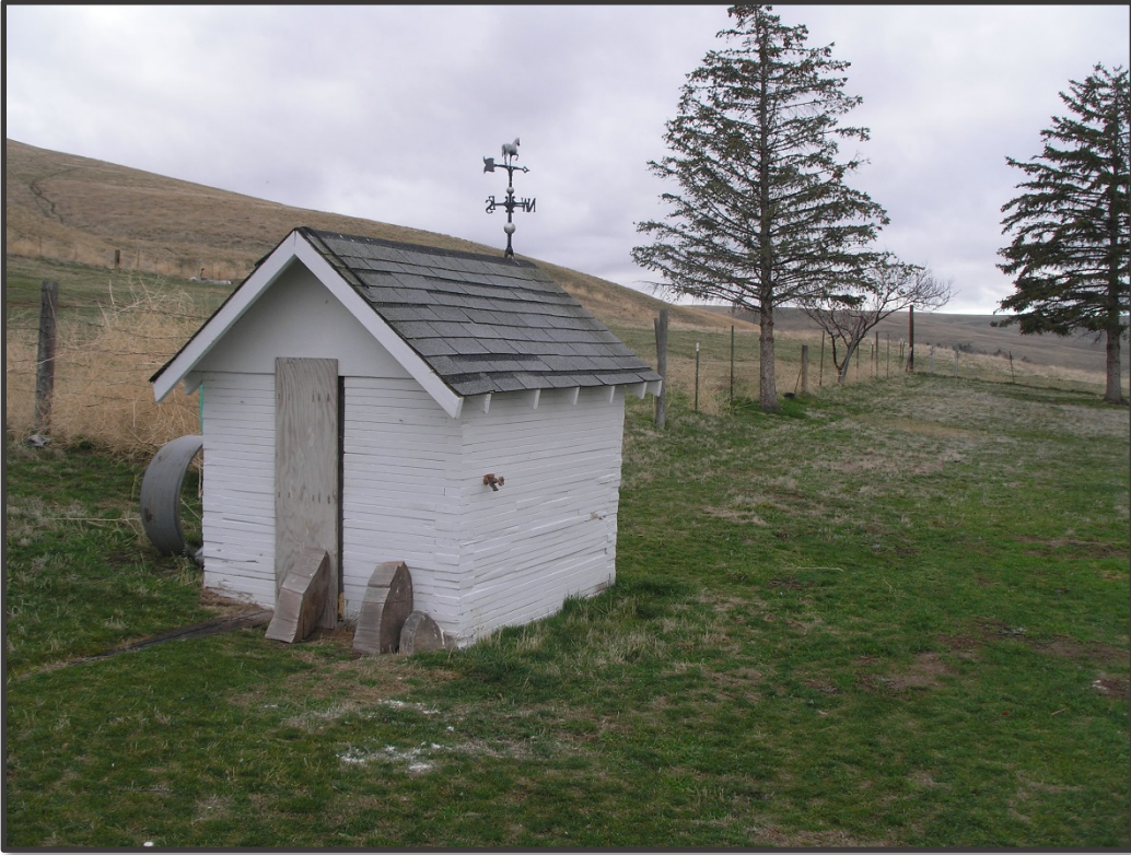
Pump house that will supply potential off-stream water.
