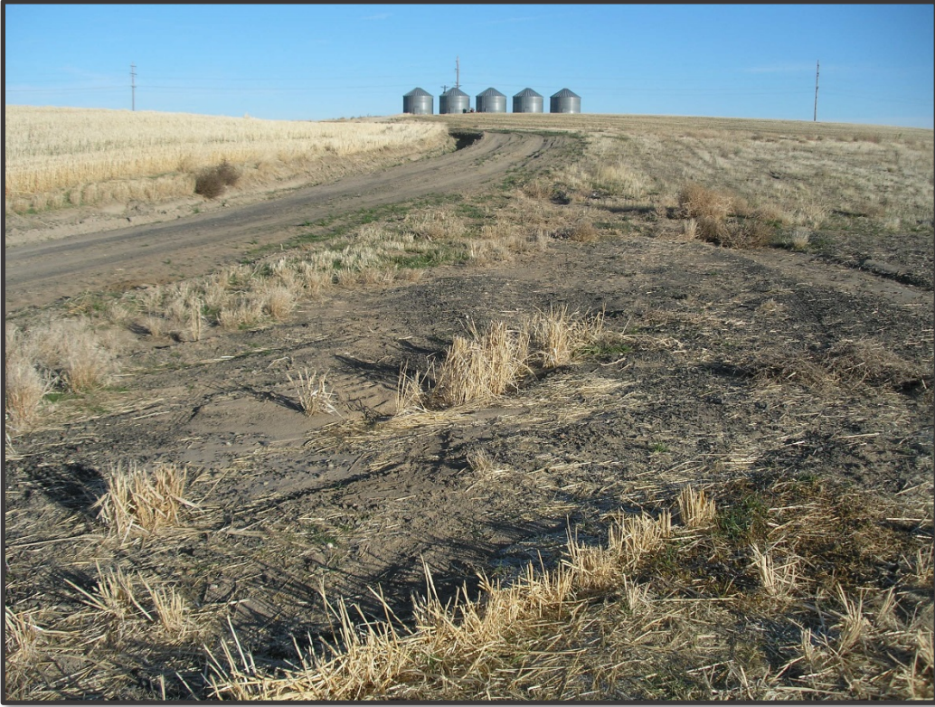
Eluvial fan deposit in a field of the access road from high water event.
