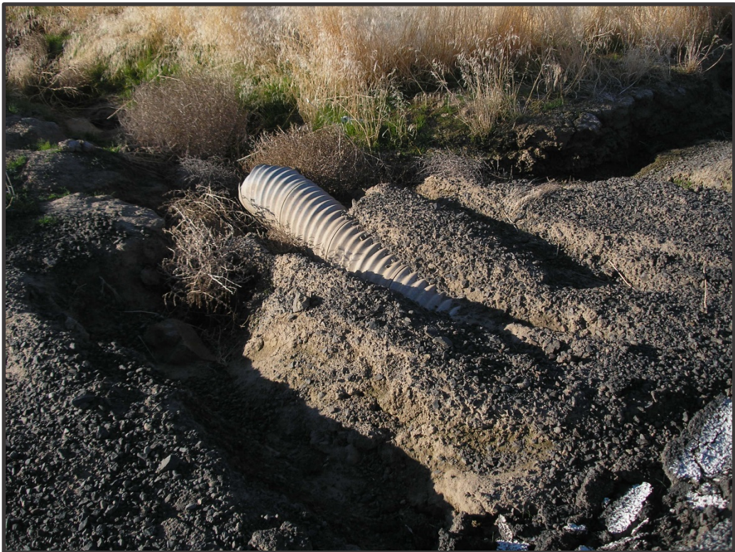
Culvert outlet on the South side of Baseline Road.
