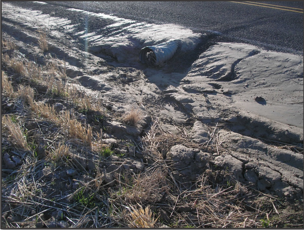
Culvert inlet on the North side of Baseline Road.
