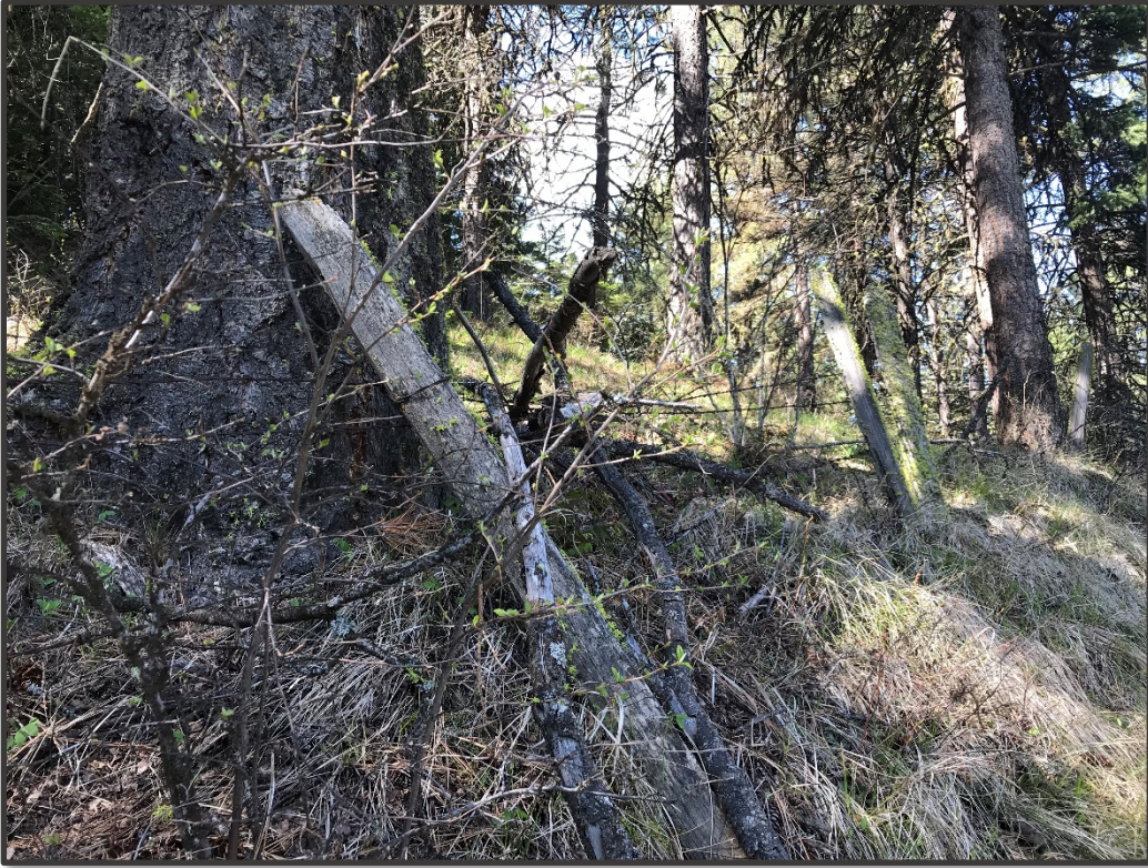
Dilapidated cross-fence that would be replaced.
