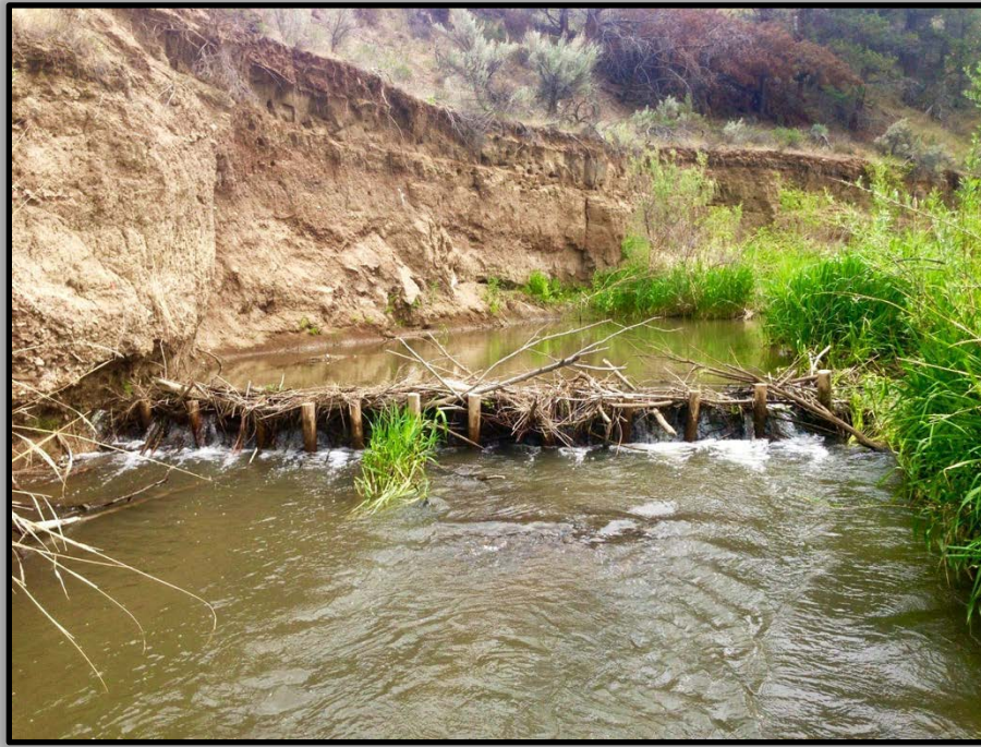
Example of BDA from Bridge Creek in Wheeler County, OR to be installed in Morrow County.
