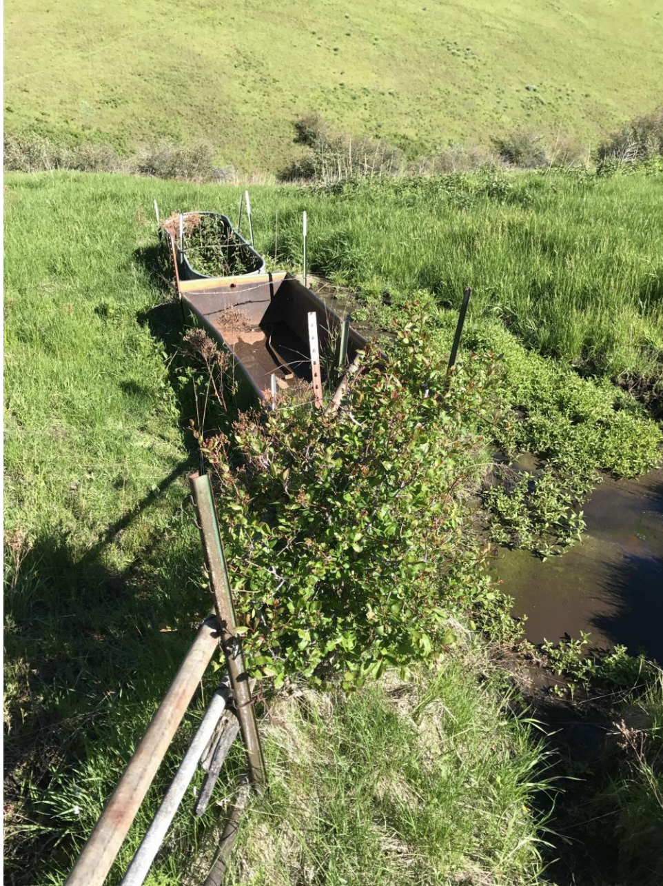
Spring Source #2 and troughs: Dilapidated troughs at spring site #2. New troughs will replace these derelicts. Spring source #2 is right next to troughs.
