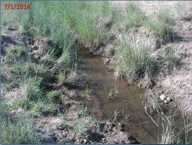
Images of existing ditch that will be piped.
