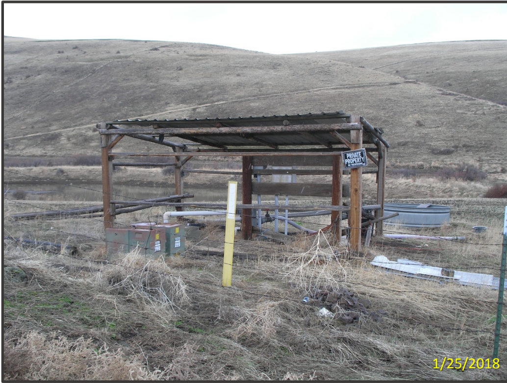
Barber existing well site (Southernmost end of project area).
