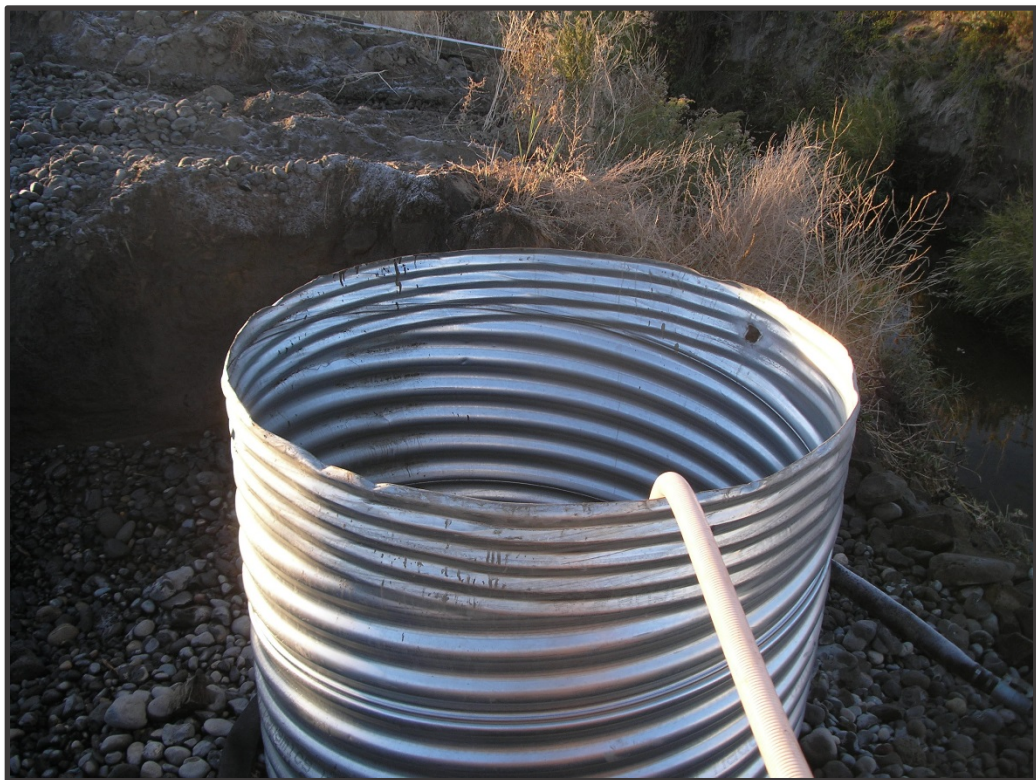
Existing sump where proposed VFD will be installed.
