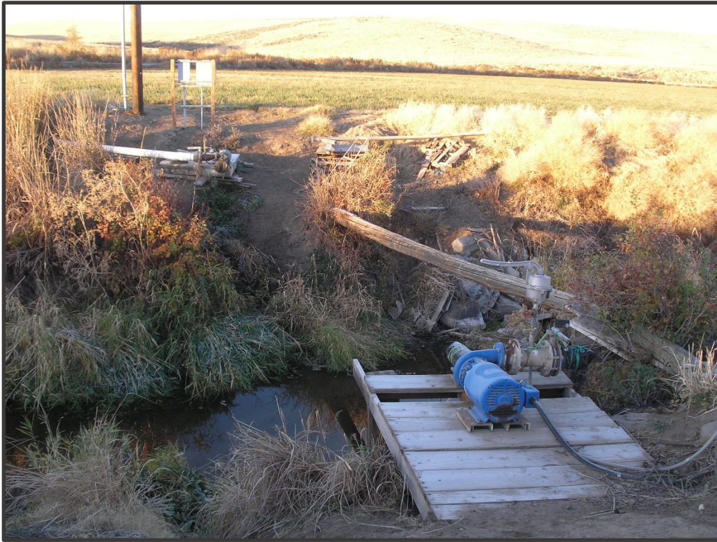
Location downstream where two pumps will be removed.
