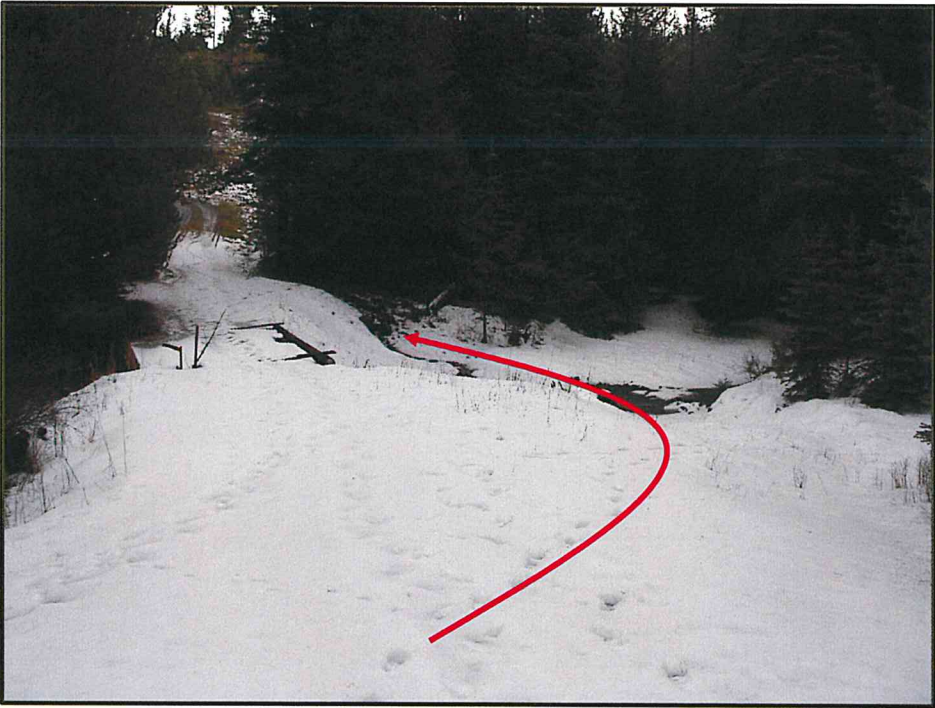
View showing where vehicles have driven to the right of the bridge and through Johnson Creek
